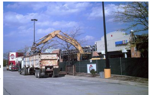
Demolition of a strip mall. Photo Credit: Clean Wal-Mart .
