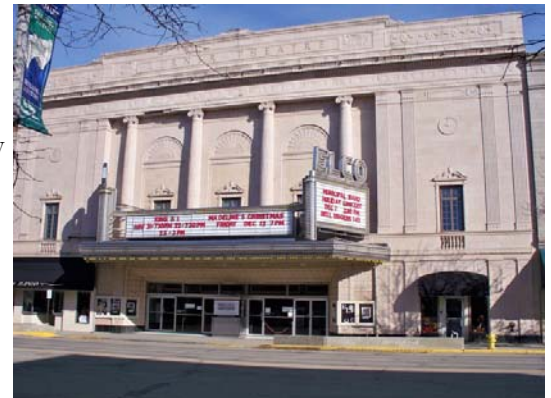
The historic Lerner Theatre in Elkhart, Illinois before the renovation efforts began. Photo credit: NowPublic .
